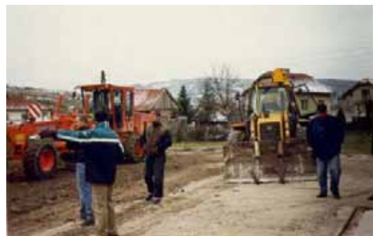
Work on the sport field in village Haljinići, Kakanj.
